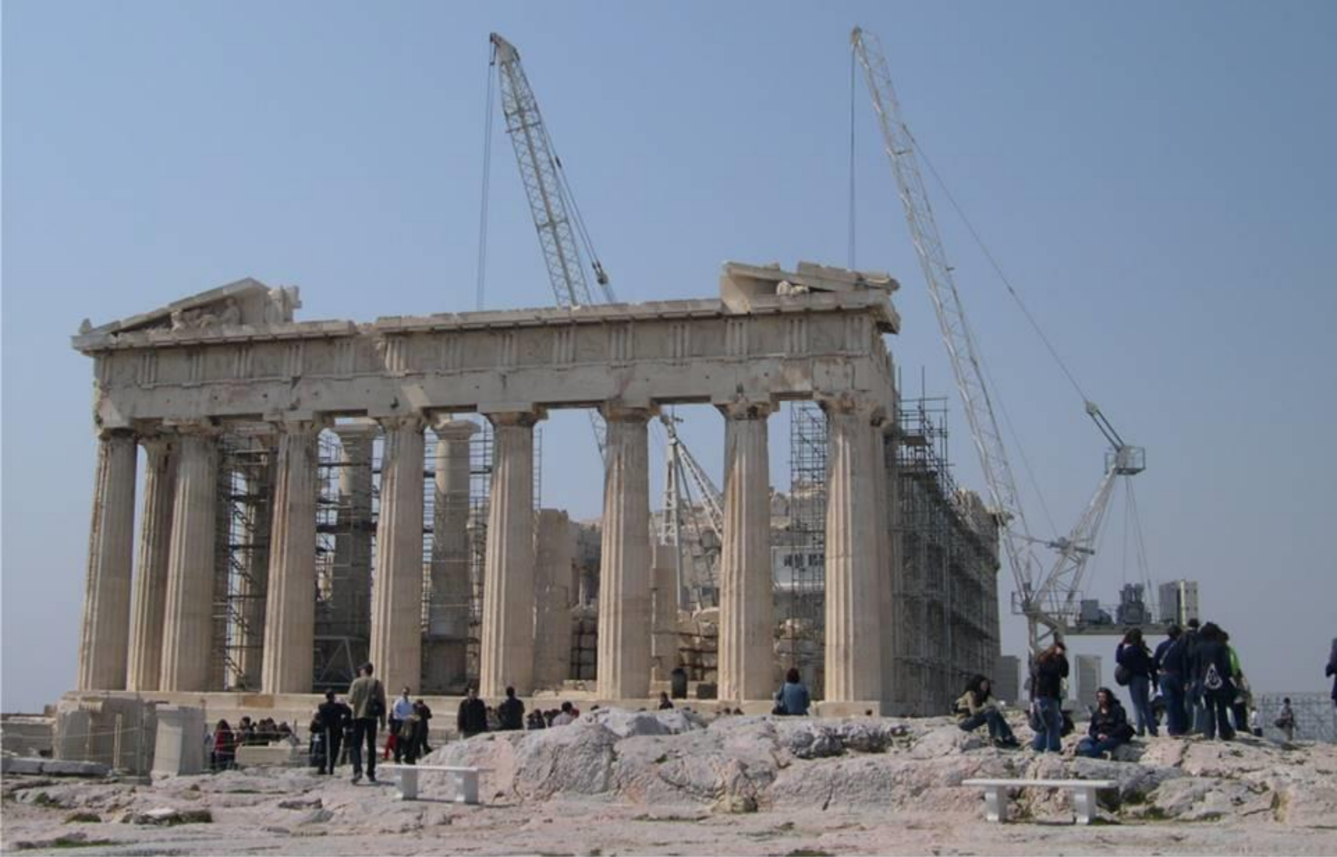
The Parthenon (circa 432BC ) under repair in 2008 - East facade
